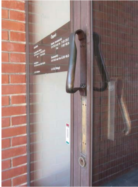
FIGURE 3 Photograph taken in the building of the Architecture Department, Aalto University, Otaniemi Campus, showing where a door handle has been removed.
