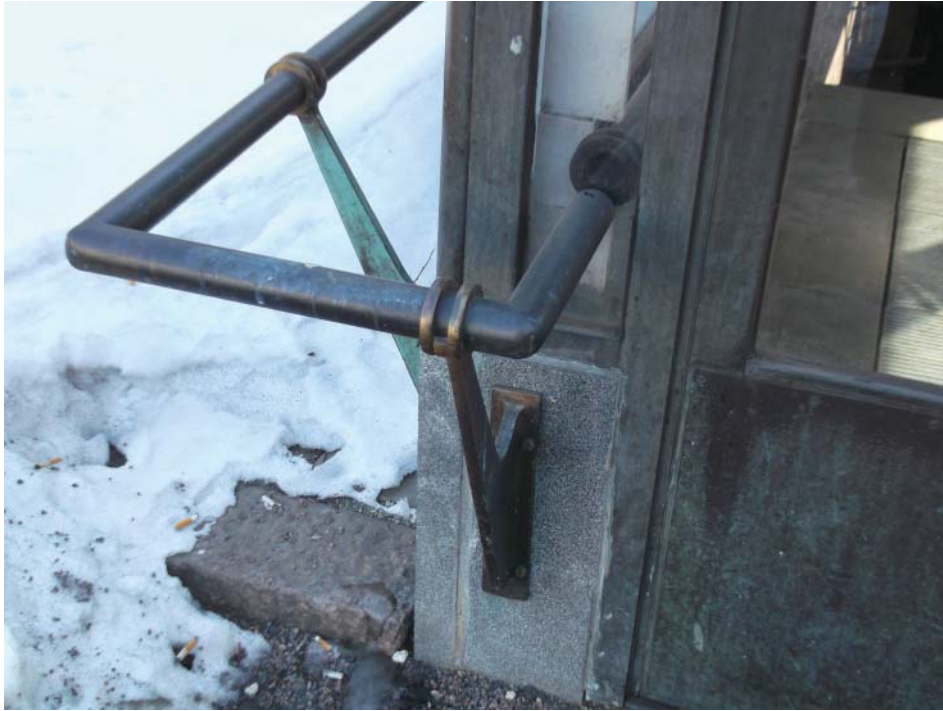
FIGURE 2 Photograph taken in March 2013 of the replacement rail support in place at the Erottaja Pavilion.
